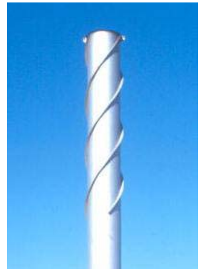
This eddy shedding structure on the stack has no real effect on dispersion from the stack.
