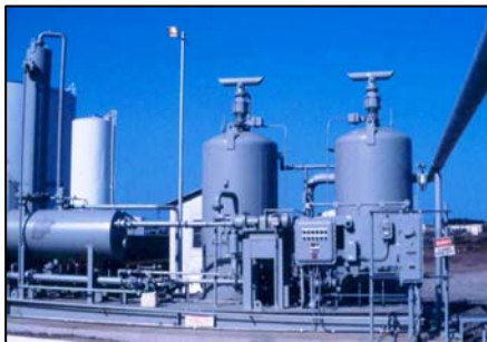
Dual adsorbers for capturing petrol vapours
