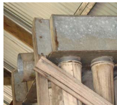
Close up of the bag filter from a gold mine
