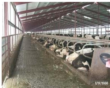
Flushing drain in free-stall dairy
