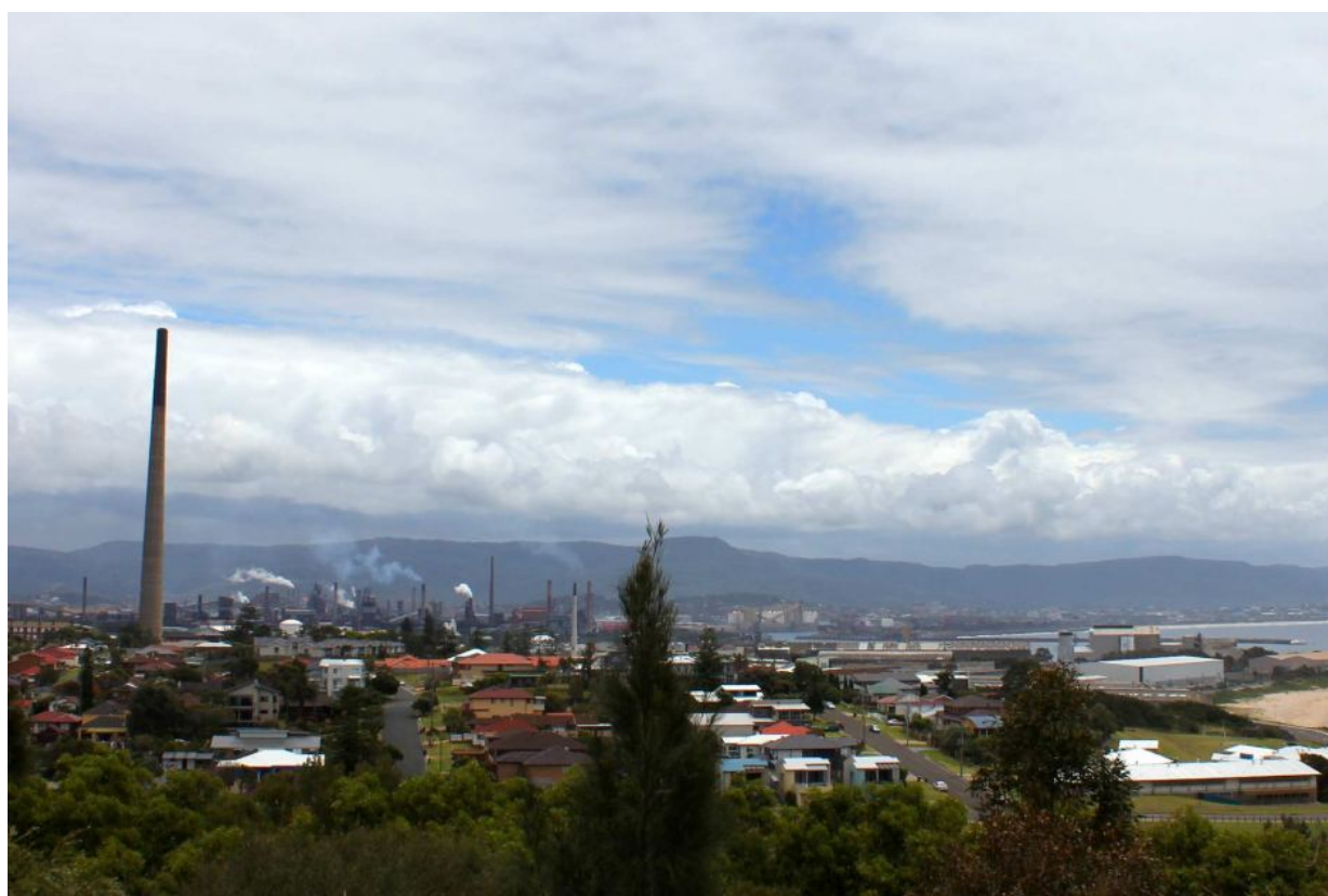
Figure 6 The stack at Port Kembla before demolition in 2014 (ABC, 2015).
