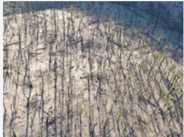
The area was inspected with drone due to ongoing safety concerns regarding walking in the area.
