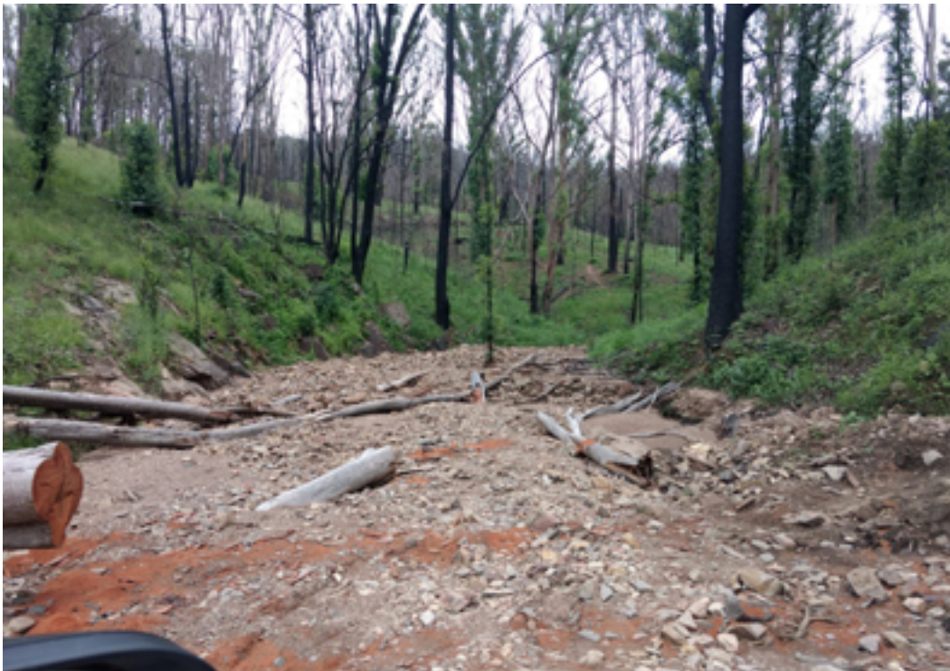
Figure 5: Mid North Coast fire-affected landscape following heavy rains. In this image: sediment from erosion backed up in a blocked road drainage structure, demonstrating the potential for erosion in post-fire environment. Effects such as this will have been quite widespread across NSW fire-affected areas on both public and private land.
