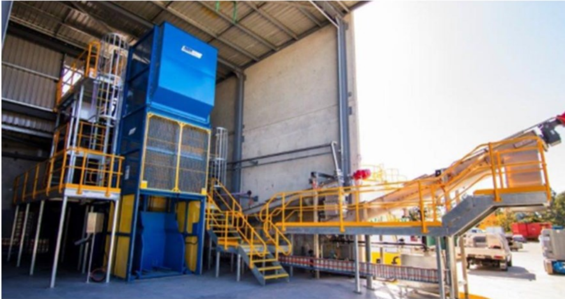
Figure 28: Cleanaway HazPak II located at St Marys, NSW
