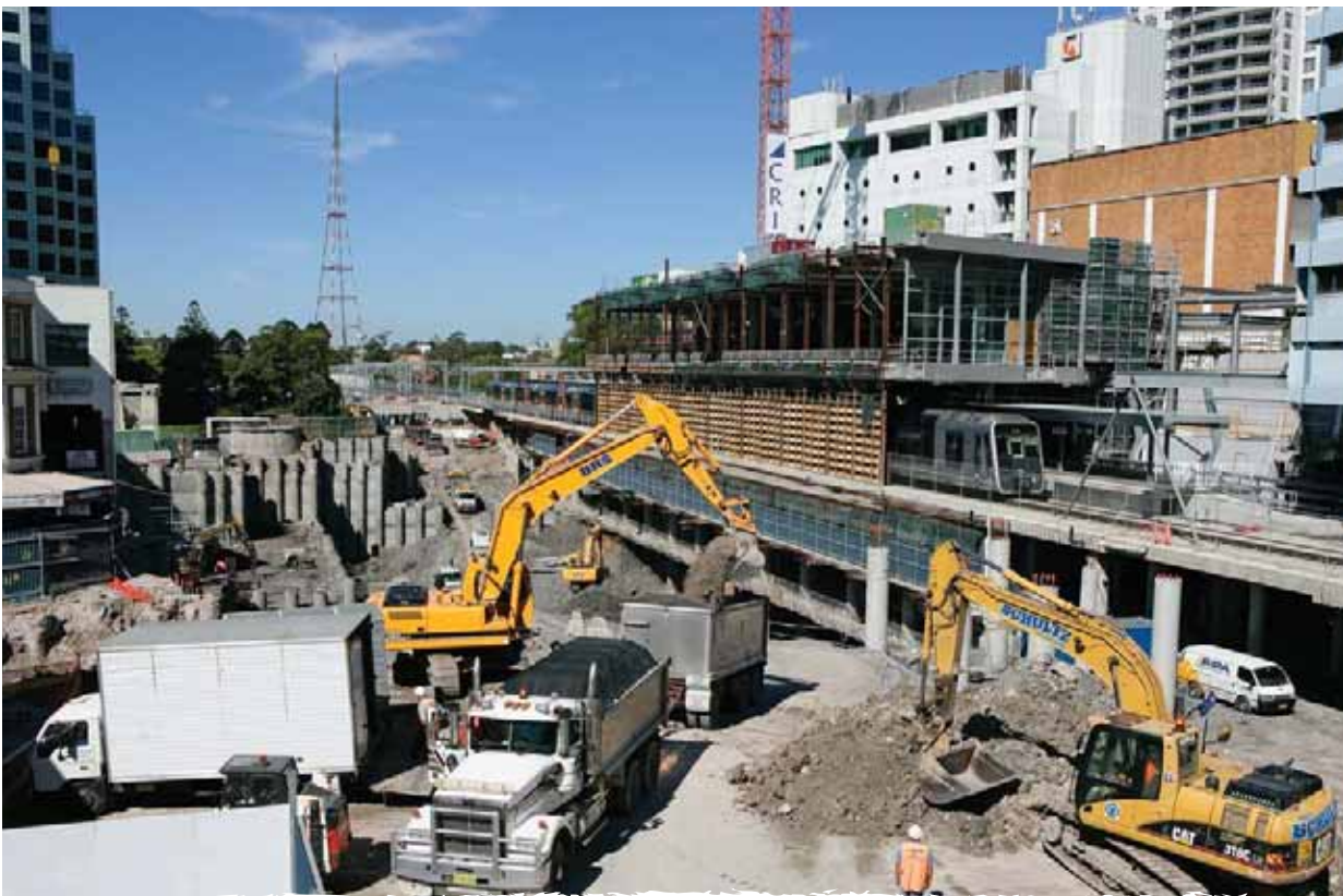
A quantitative assessment usually suits complex works (Transport Infrastructure Development Corporation)
