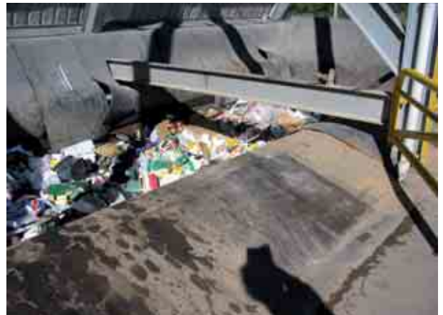
Photo 30.22 Retrofit of platform edge to support movement of site plant
