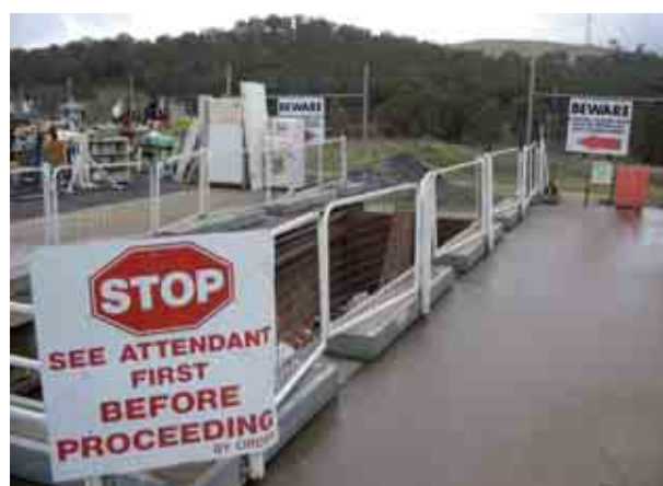
Photo 31.2 Signage and safety barriers surrounding the general waste skip bin
