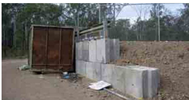
Photo 33.1 Transfer station platform
