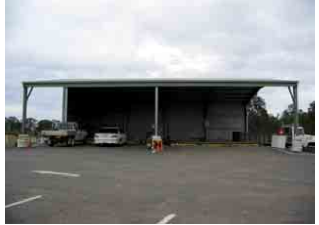
Photo 32.2 Mixed waste drop-off point
