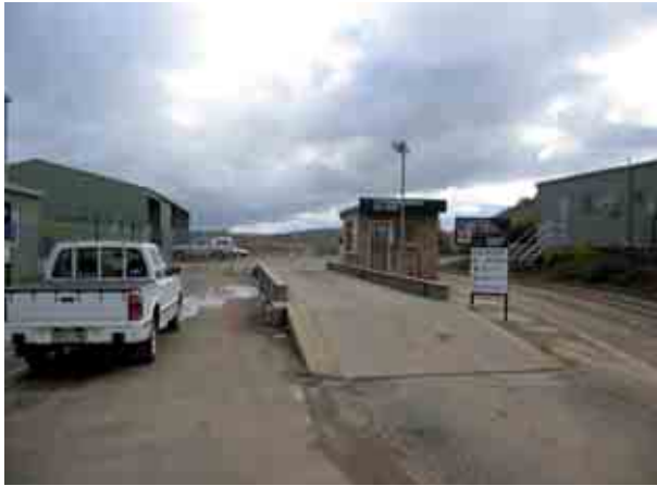
Photo 28.3 Site entry via a single lane weighbridge and gatehouse
