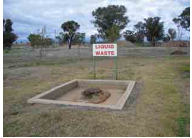
Photo 27.15 Signage at liquid waste area (Note: Liquid waste should be stored in a covered and bunded area)
