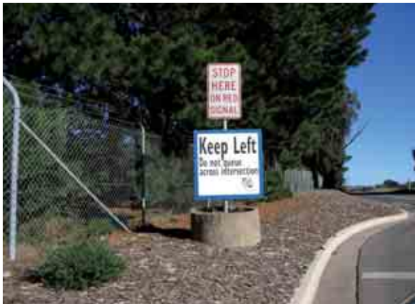
Photo 30.3 Signs outside site entrance used as part of the traffic control system
