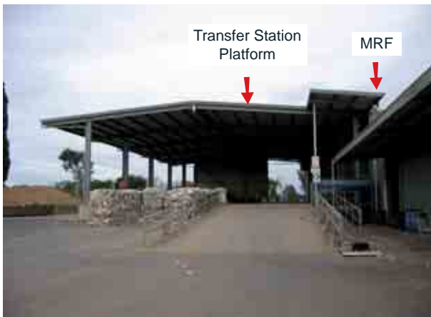
Photo 34.5 Transfer station platform and MRF
