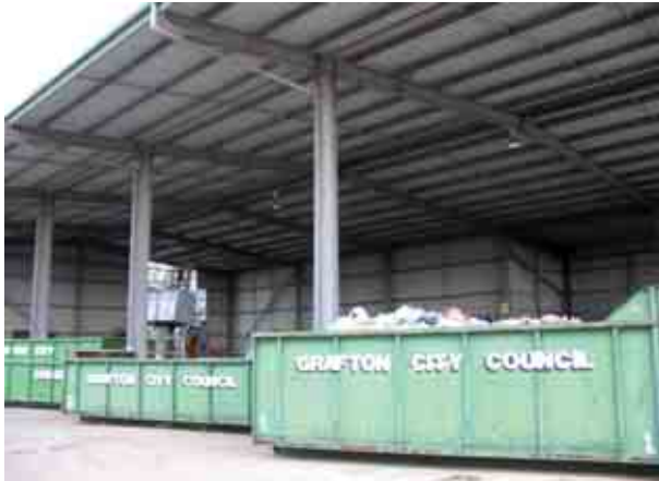
Photo 34.4 Cover over skips
