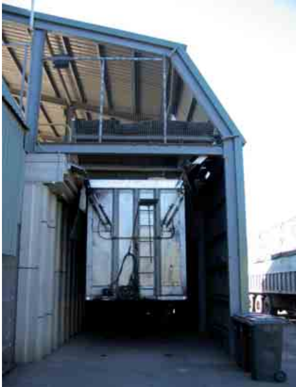
Photo 30.7 View of transfer trailer from the base of the platform
