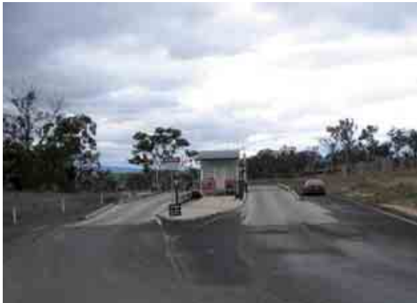
Photo 36.1 Double lane weighbridge and gatehouse
