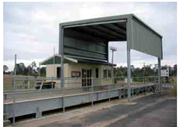
Photo 32.7 Cover over weighbridge
