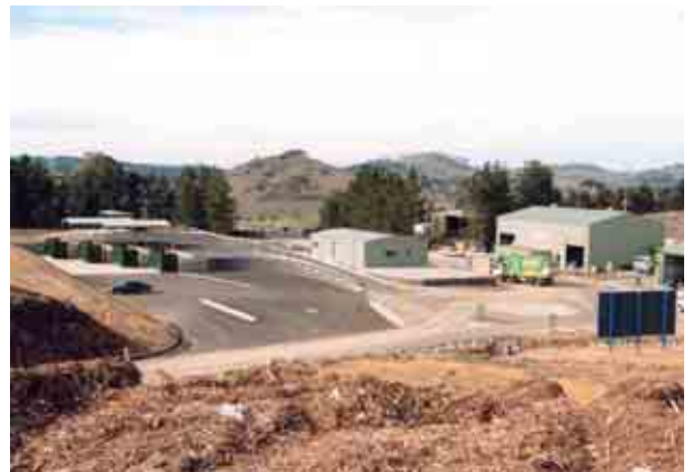
Photo 28.6 View of the site entrance and transfer from the landfill
