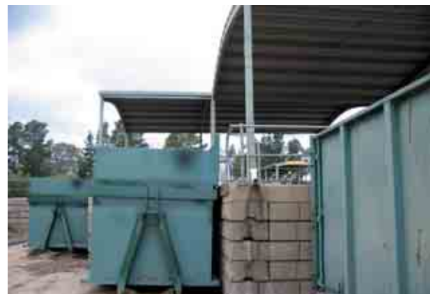
Photo 28.11 Waste transfer station platform, roof and skip bins
