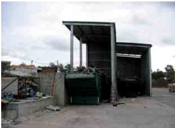
Photo 35.5 Double-shelter enclosure for skip bins
