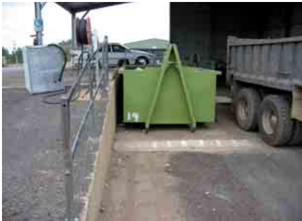
Photo 32.5 Waste transfer platform
