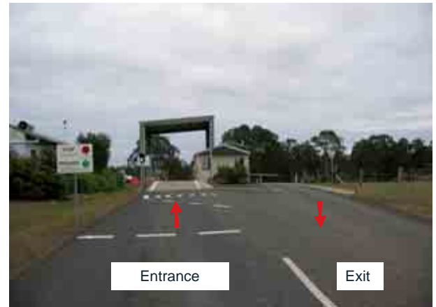
Photo 32.6 Site weighbridge and gatehouse
