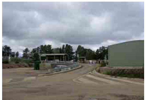
Photo 28.7 Transfer station, waste oil and reuse centre
