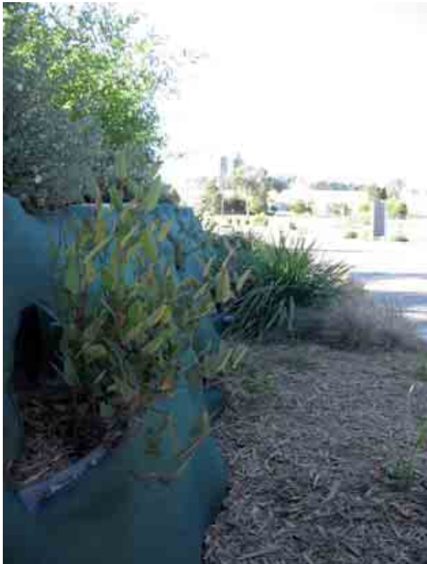
Photo 30.23 Retaining wall made from recycled tyres and planted with vegetation
