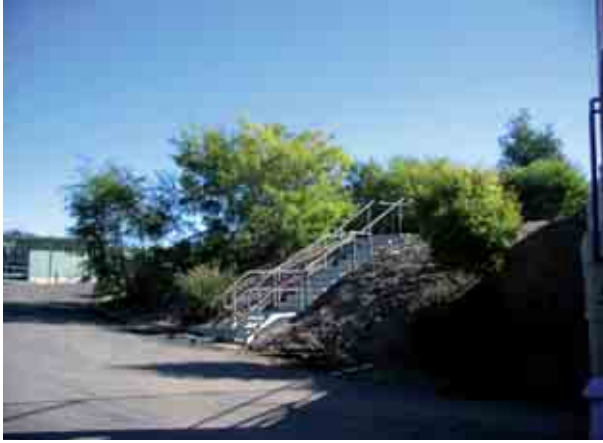
Photo 30.26 Landscaped batter adjacent to transfer platform
