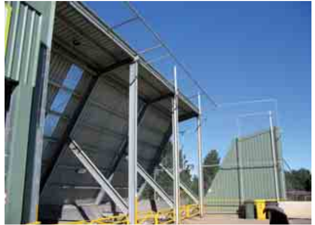
Photo 30.12 Wind-break and cover over large vehicles drop-off point
