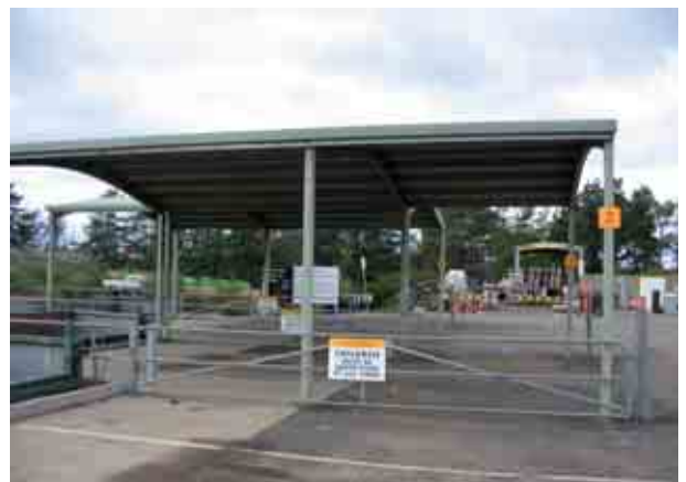
Photo 28.14 Guide rails and line markings between drop-off areas
