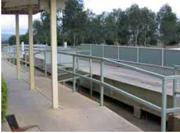
Photo 27.13 Close up of distance between site office and weighbridge
