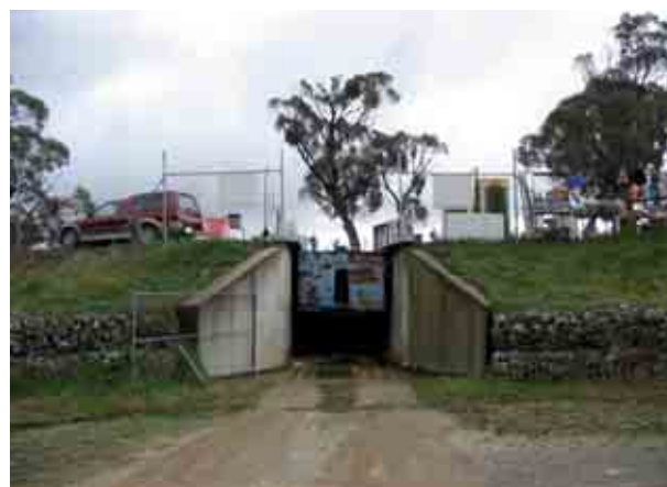
Photo 31.3 Natural topography used for transfer platform
