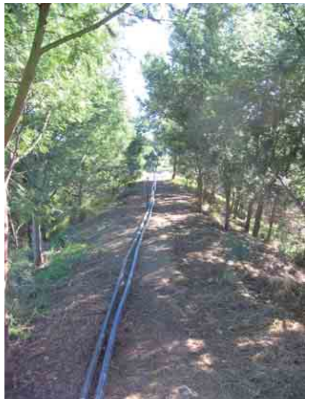
Photo 30.25 Vegetated mound on western site border
