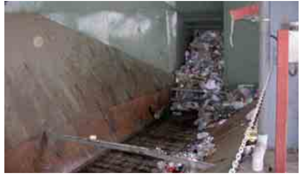
Photo 34.7 Conveyor used to feed recyclables into MRF
