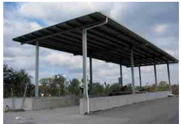
Photo 37.2 Kempsey transfer station (view from rear)
