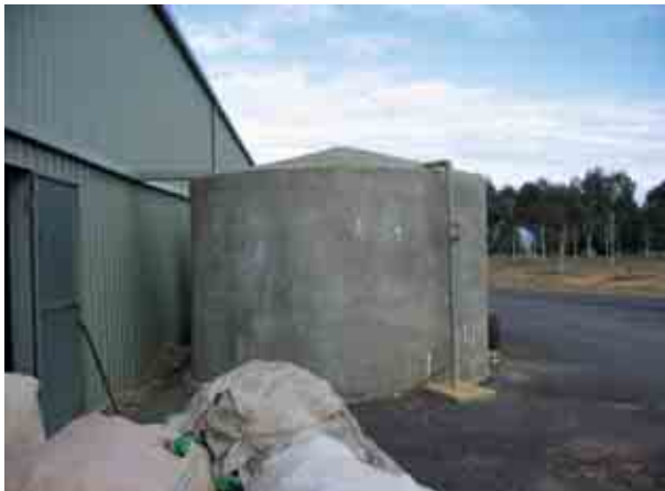
Photo 27.8 Cement rain water tanks behind the MRF and reuse centre
