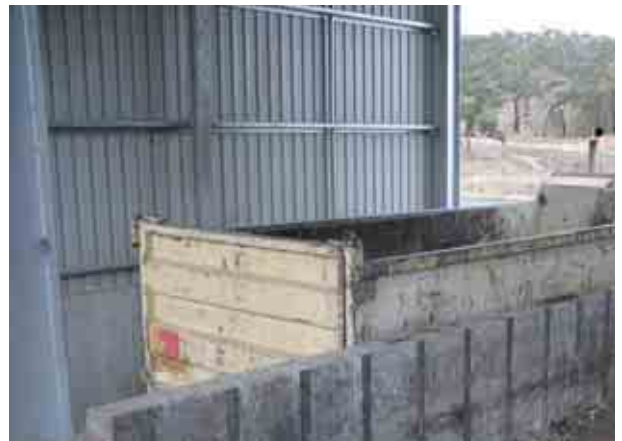
Photo 36.4 Truck waiting to be loaded at the end of the push-pit
