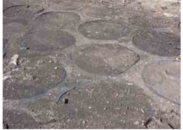
Photo 30.24 Recycled tyres to provide additional support for vehicle movement
