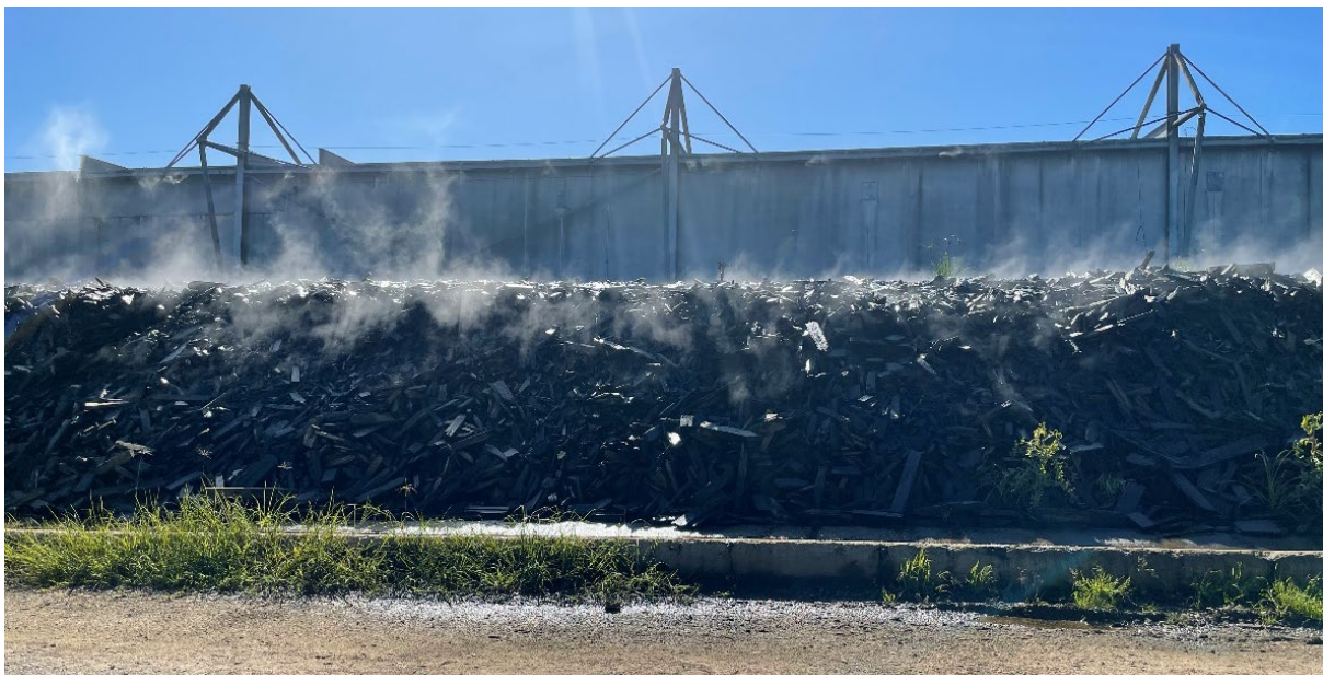
Figure 16 Active biofilter
