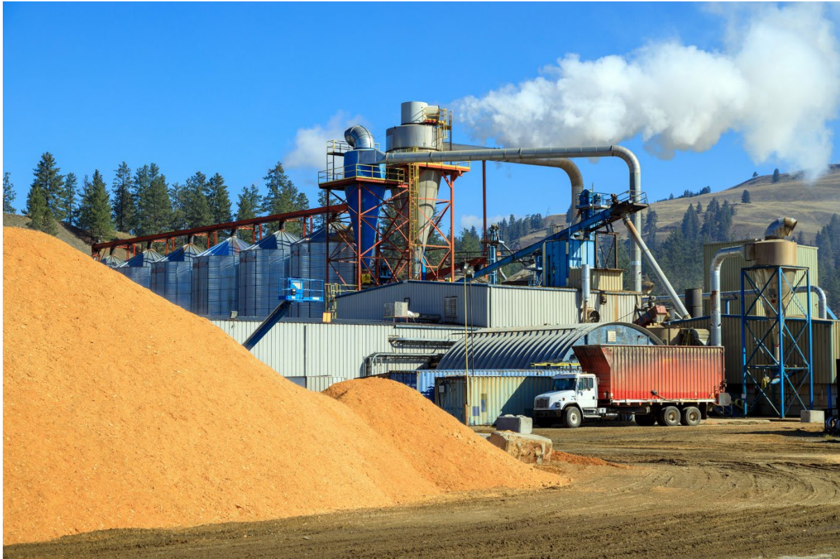
Figure 4 Example of a dust collection system at a sawmill
