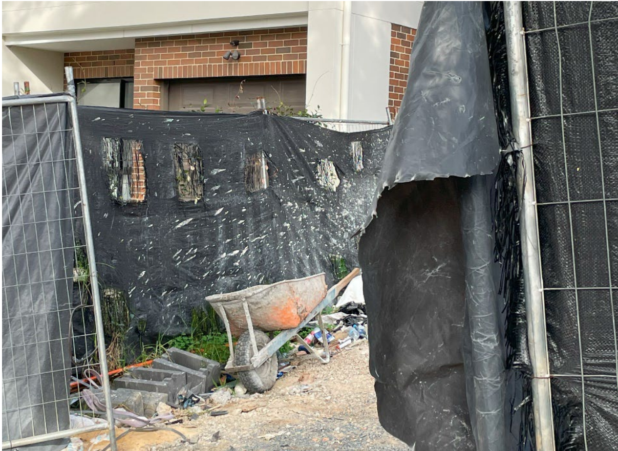
Figure 7 Example of porous shade cloth with additional openings for high wind events Source: Jane Barnett/Zephyr Environmental
