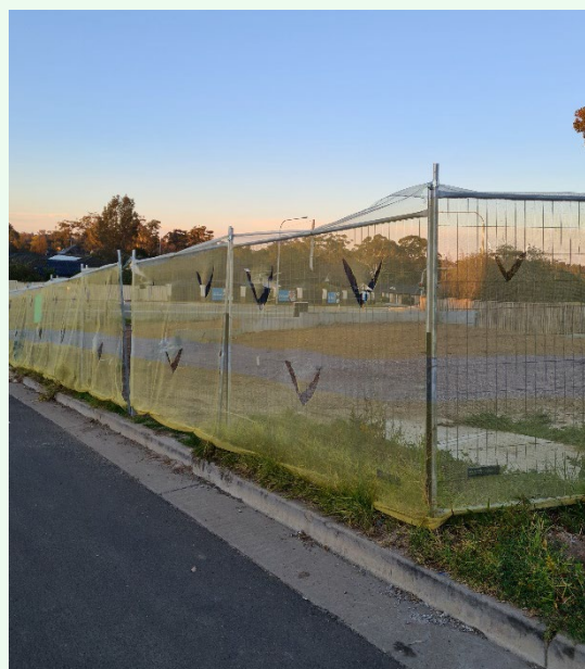
Figure 9 A fence with adequate dust screens
