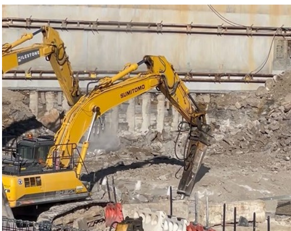
Figure 2 Dust produced from rock and cement breaking
