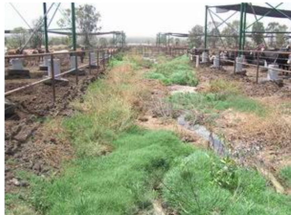
Figure 12 Poorly maintained drain
