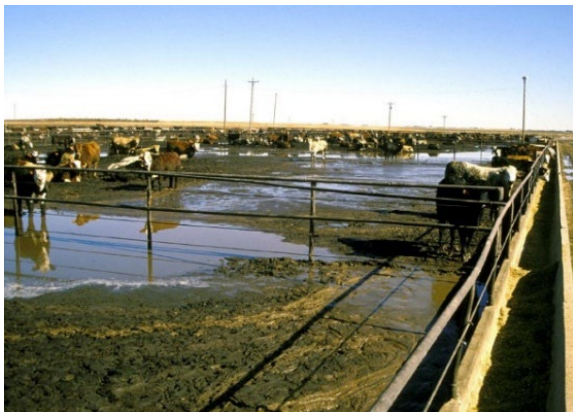
Figure 8 Drainage slope too flat to allow effective run-off
