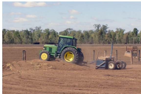
Figure 5 Manure mounding using a box scraper Source: Tucker et al. 2015
