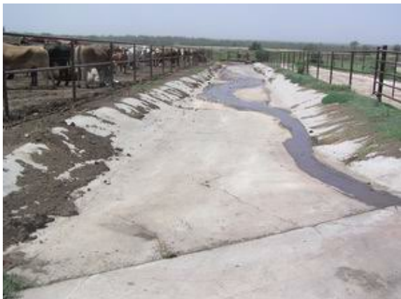
Figure 11 Well constructed and maintained concrete drain
