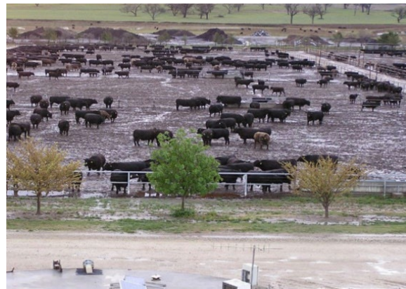
Figure 9 Poor design with pen-to-pen drainage
