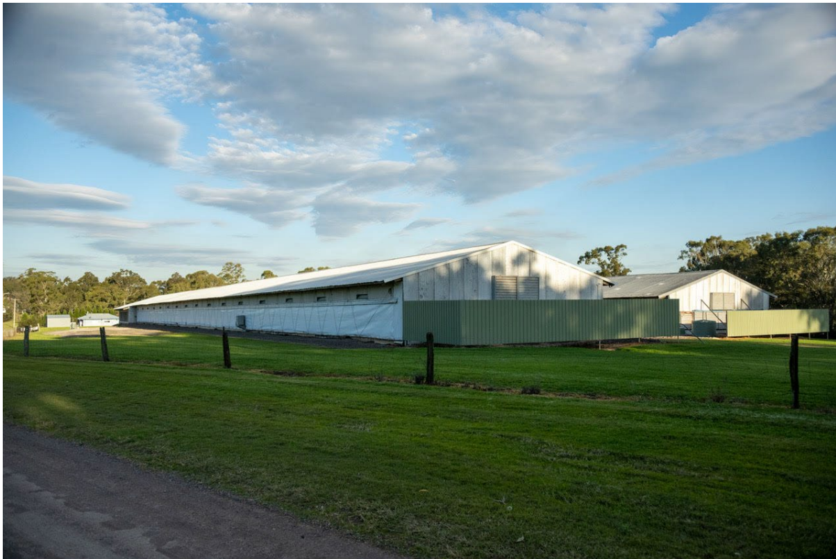
Figure 4 Example of a windbreak wall at the end of a chicken shed Source: Jane Barnett/Zephyr Environmental
