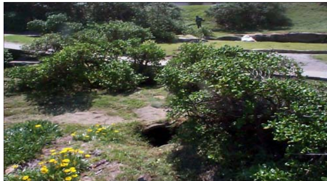
Exposed Drain prior to Enviro-media installation
