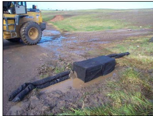
Installation of devices containing RO
