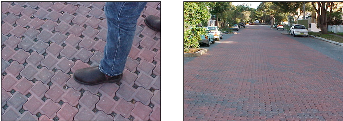
Figure 3.1. Permeable pavers installed in Smith Street, Manly to aid in stormwater management.
