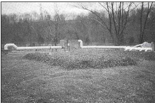
Figure 4.5. Compost biofilters remove a wide range of compounds from air at relatively high contamination rates (Alexander, 1999).
