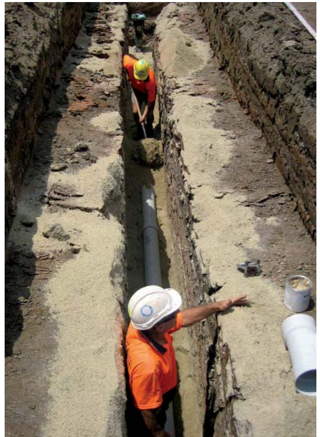
Above: 50% glass/sand blend covering the sewer pipe
