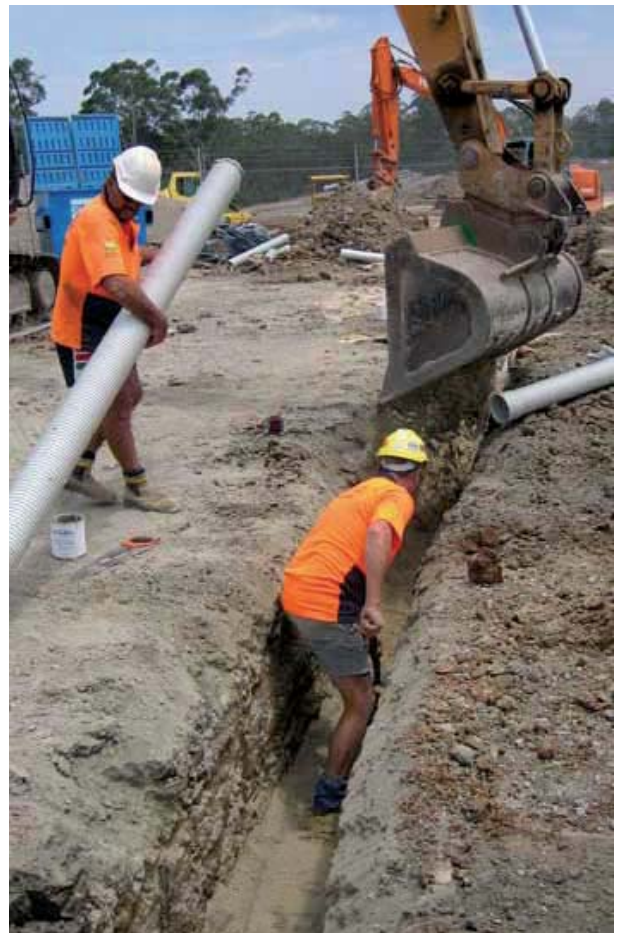
Below: 25% glass/75% sand blend sewer pipe bedding placement
