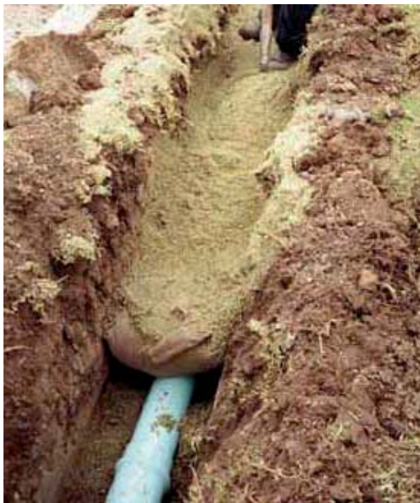
Below: 100% glass fines bedding the sewer pipe
