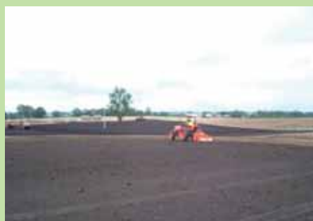
Figure 1 The 5 ha trial site after spreading of 100 mm layer of topsoil (left). Spreading and incorporation of compost (centre). After incorporation of compost and surface seeding with hydromulch (right).
