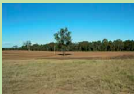
Figure 1 The 5 ha trial site after spreading of 100 mm layer of topsoil (left). Spreading and incorporation of compost (centre). After incorporation of compost and surface seeding with hydromulch (right).
