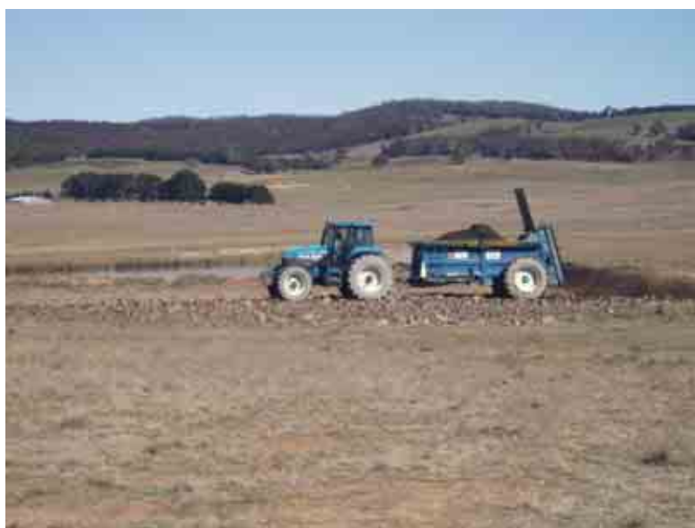
Figure 12. A chain driven spreader was used to apply the composted soil conditioner and mulch to a depth of 25-30 mm.
