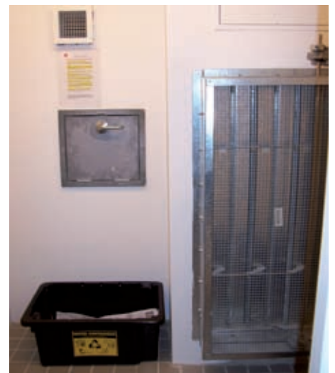
Court block service compartment
