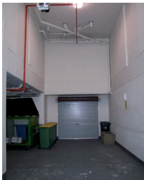
Elevated ceiling height to allow for front-lift waste collection if needed
