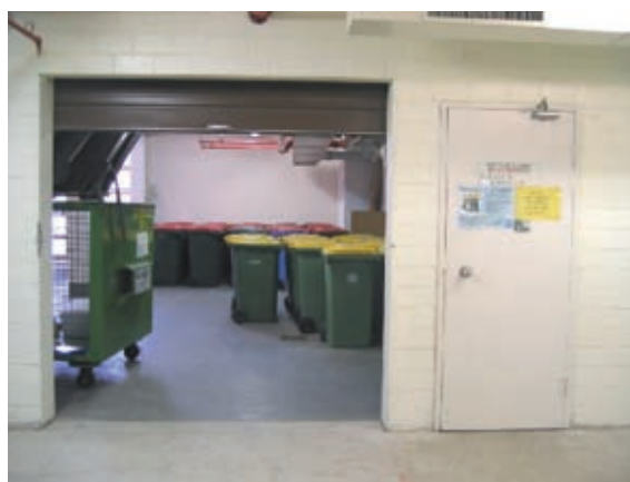
Access to the central storage and collection room from the carpark
