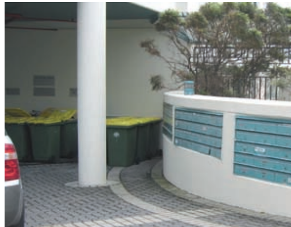
Recycling bins stored adjacent to resident mailboxes
