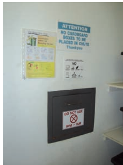
Signage in service compartments of the tower
