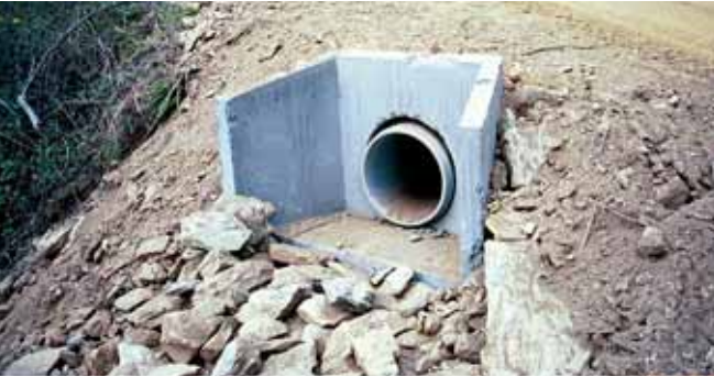
(b) Artificially rocked surface
