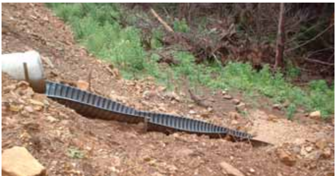
Figure 5.17: Drop-down structure and dissipater
