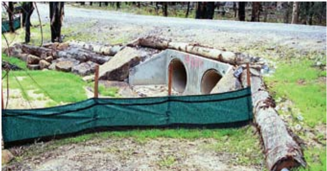
(a) Establishing groundcover
