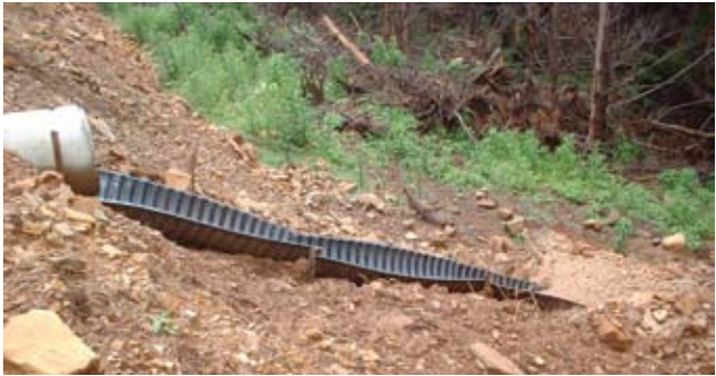
Figure 5.17: Drop-down structure and dissipater
