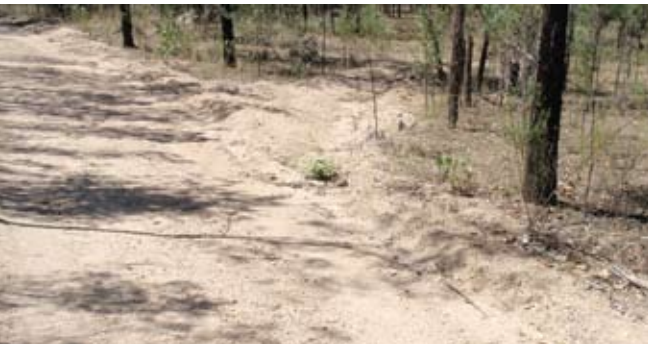
Figure 5.9: Mitre drain
