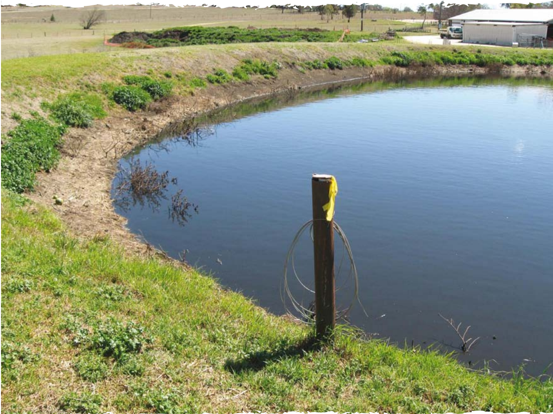
This pond has sufficient residual capacity to store effluent during wet-weather conditions (photo: M Hatzakis/DECCW)
