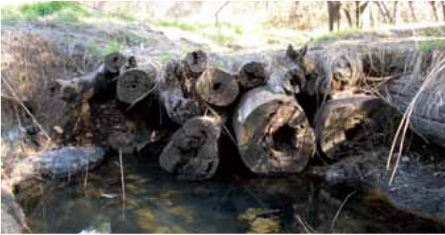
Figure 5.22: Gully stuffer
