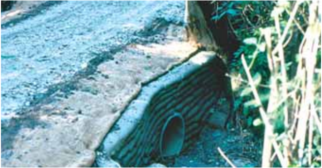
Figure 5.20: Culvert crossing
