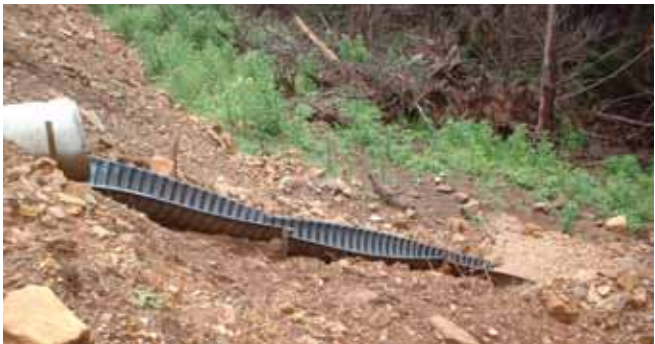
Figure 5.17: Drop-down structure and dissipater
