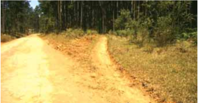
Figure 5.9: Mitre drain
