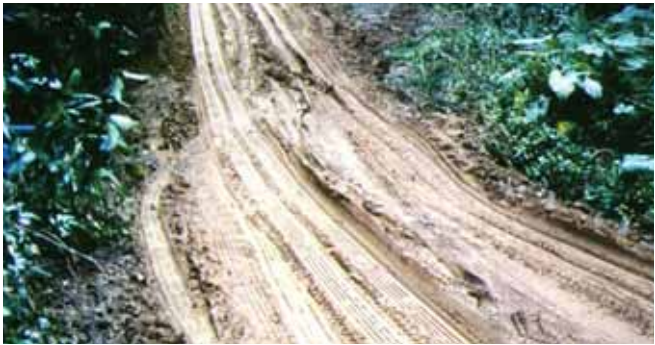
Figure 5.26: Example of road surface breakdown
