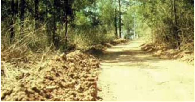
Figure 5.14: Earth windrow
