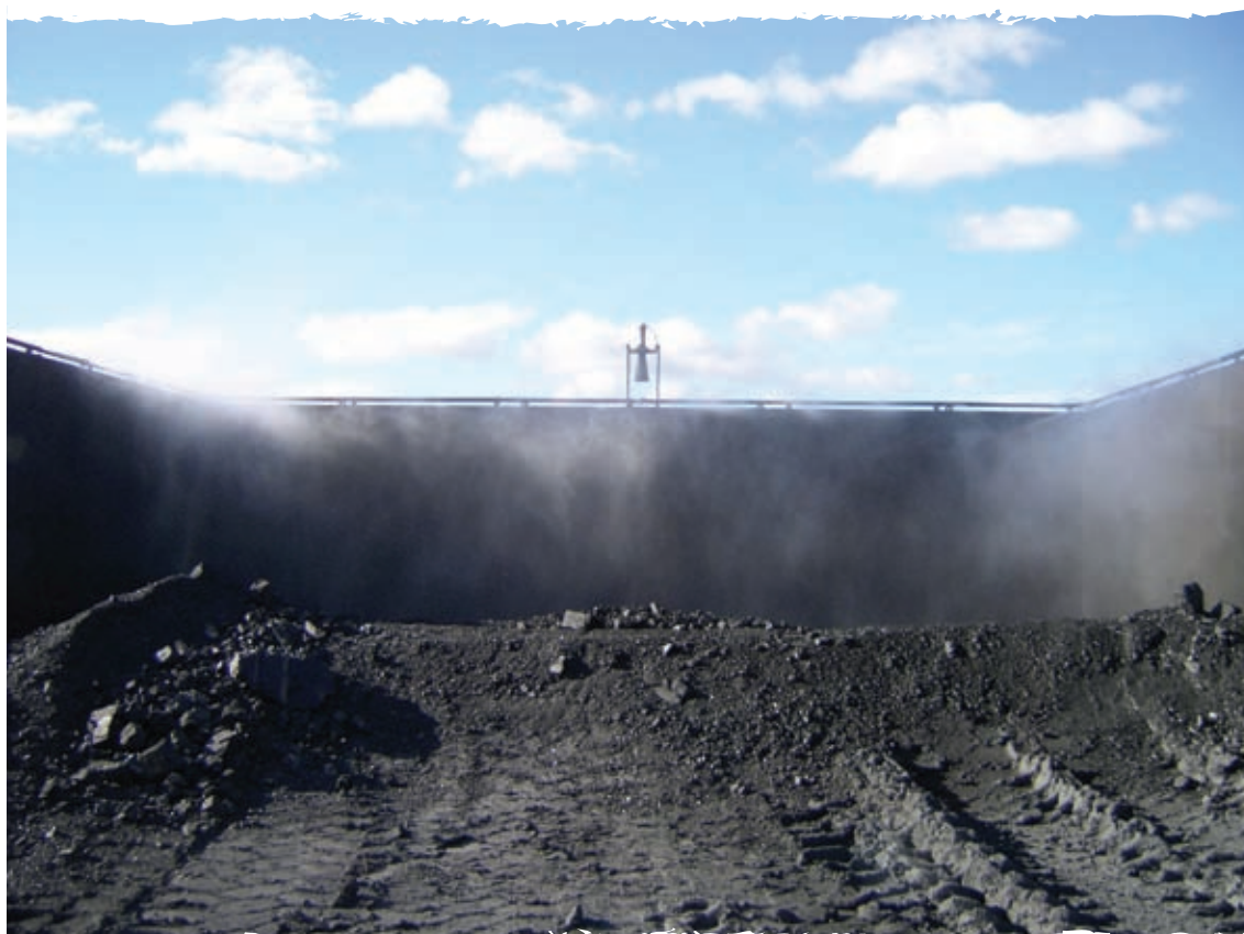
Automated sprays are used at a ROM hopper to reduce fugitive emissions (photo: B Green/DECCW).
