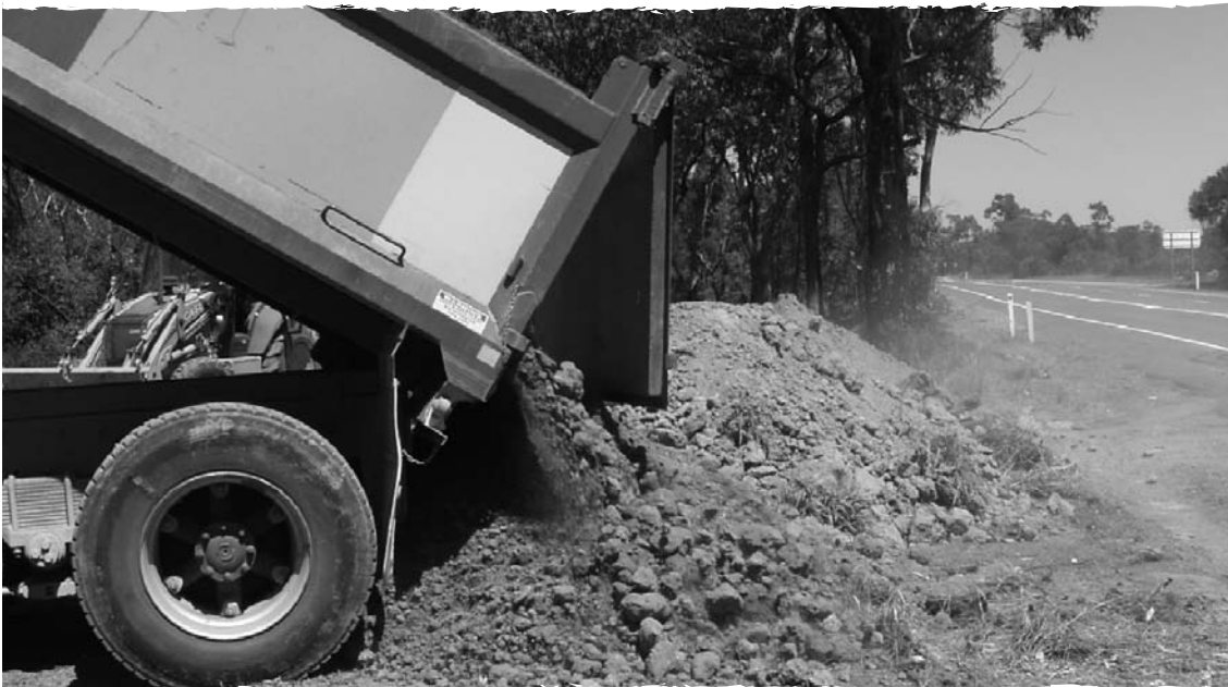
Earth mounds being created to prevent access to land.
