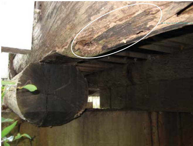
Figure 1: Sapwood which had not been preservative treated, decaying after a few years in service
