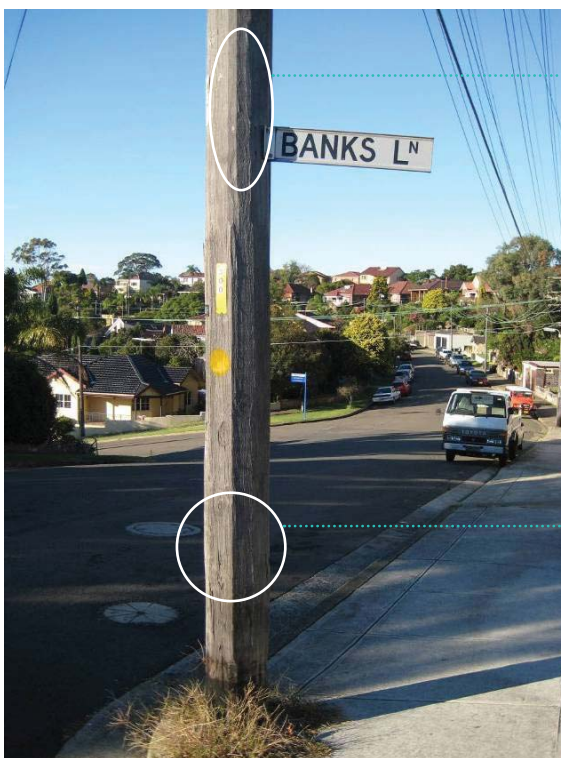
Figure 2: Desapped power pole – Sydney
