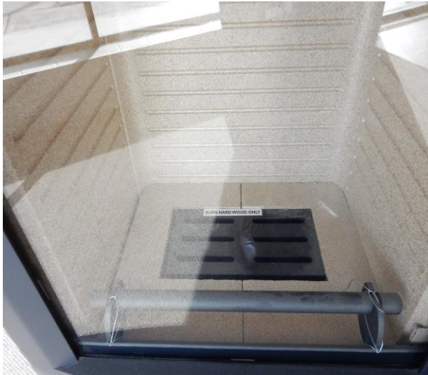
Figure 11: Fuel type plates not considered 'easily visible' (the left photo shows plate attached to the inside of heater door; the right plate is attached on the back of the heater) (Photo: Nuwyy Ly, EPA)
