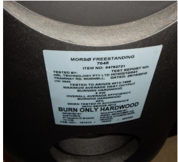
Figure 11: Fuel type plates not considered 'easily visible' (the left photo shows plate attached to the inside of heater door; the right plate is attached on the back of the heater) (Photo: Nuwyy Ly, EPA)
