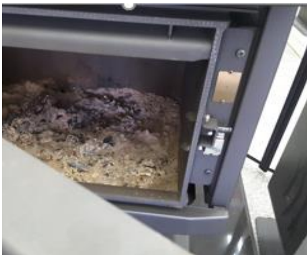
Figure 10: Fuel type plates where the wording is not visible after short use of wood heaters (Photo: Antonia Curcio, EPA)
