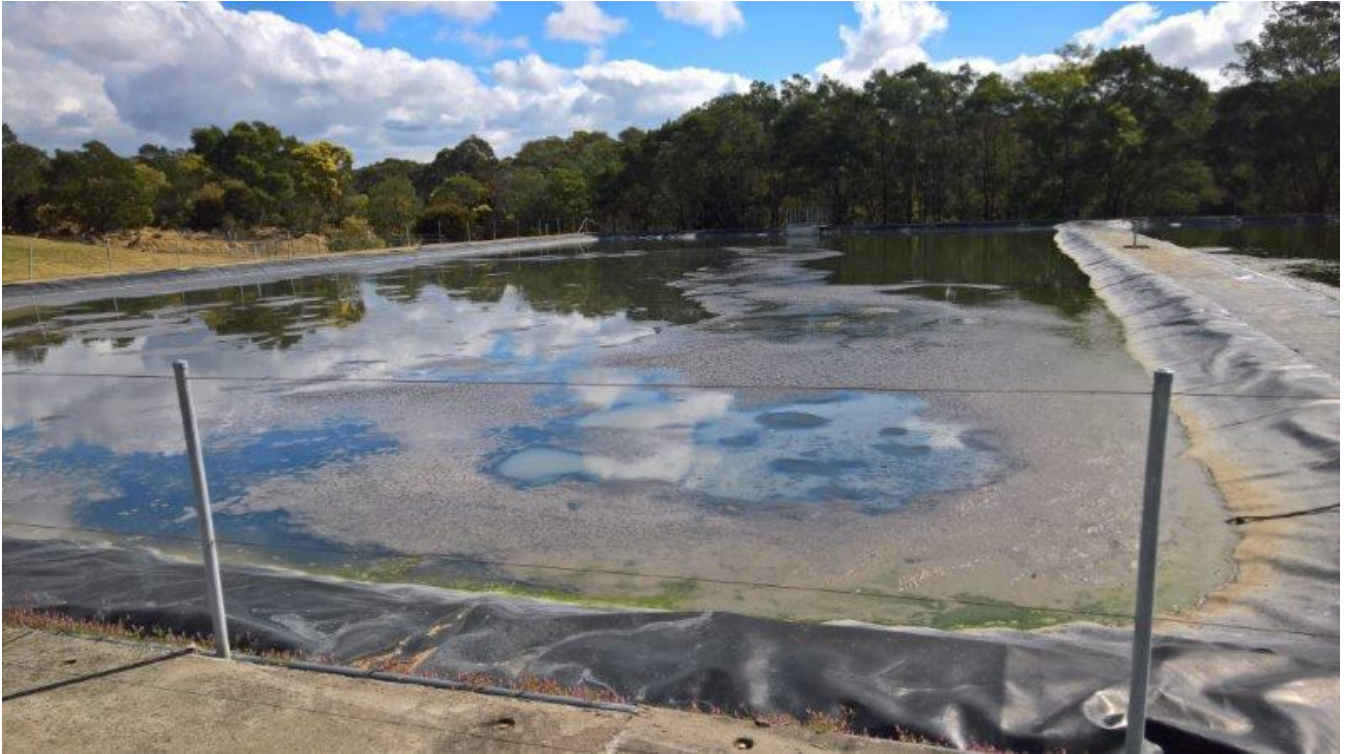
Photo 5: Fully lined sludge lagoon
