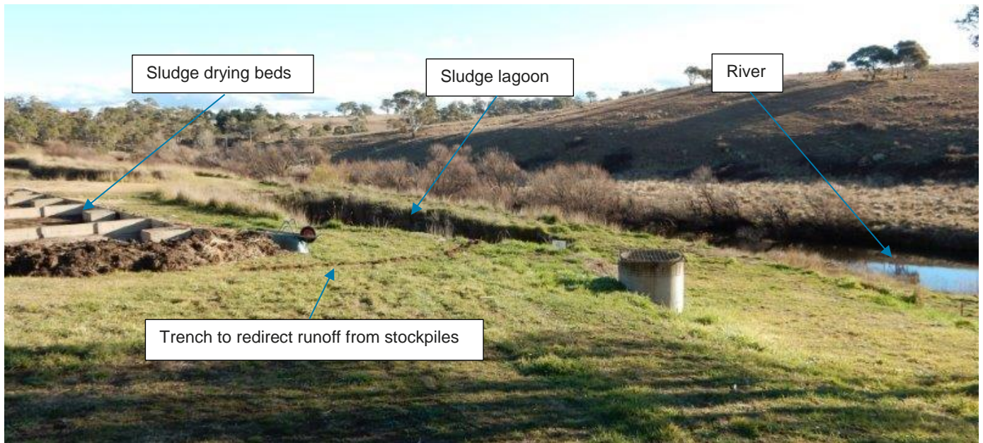
Photo 16: Sludge management adjacent to river (risk of water pollution)
