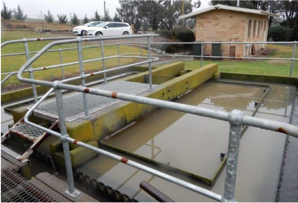
Photo 3: Primary sedimentation tank
