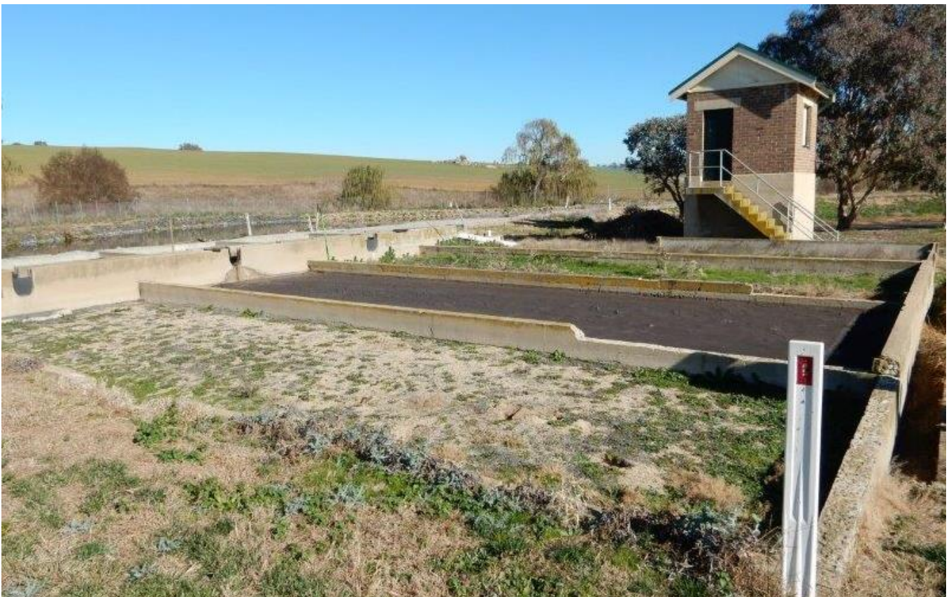
Photo 6: Sludge drying beds
