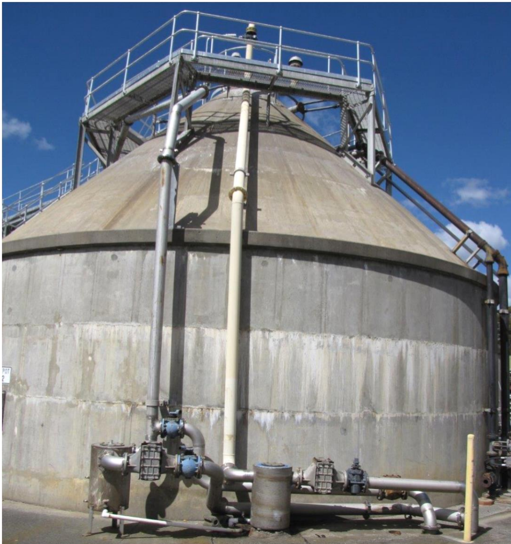
Photo 4: Sludge digester
