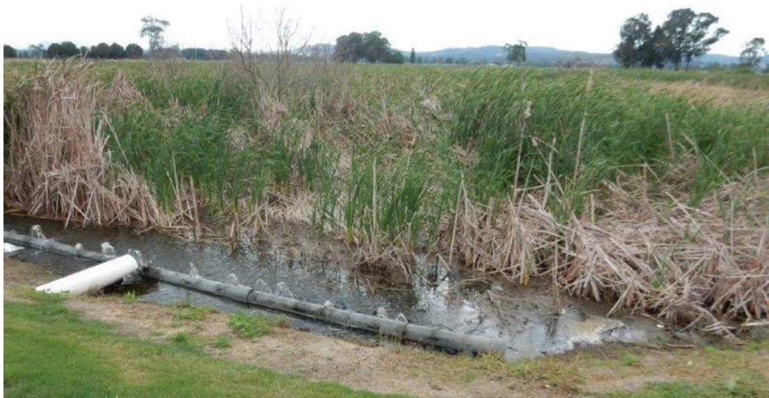
Photo 13: Discharge from tertiary pond into constructed wetlands
