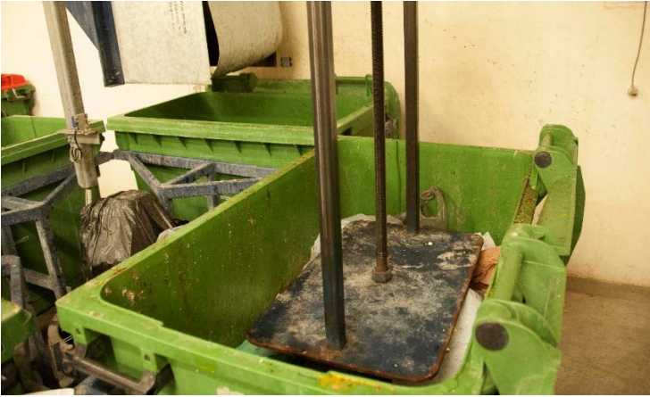
A bulk 660L bin on an automatic bin carousel with ceiling-mounted compaction (Photo: Andrew Quinn)
