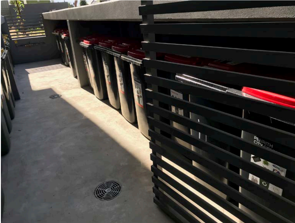
Bin storage with screening and easily accessed, clearly separated waste and recycling bins (Photo: Penrith City Council)
