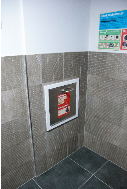
Waste chute inlet located inside a bin storage and service room on each floor of a medium-rise building (Photo: Andrew Quinn)
