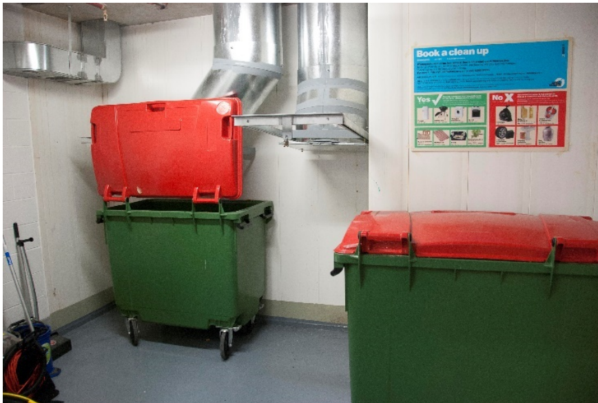
660L bulk waste bin under chute in the bin storage room (Photo: Andrew Quinn)
