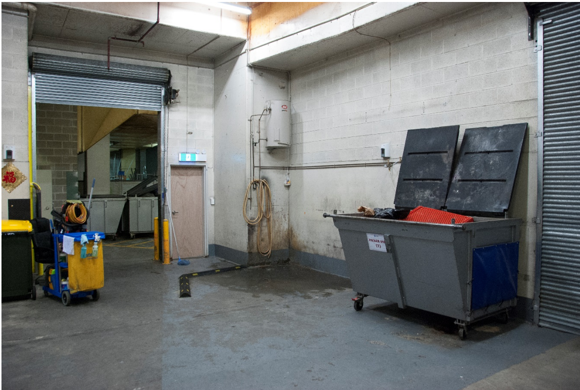
Bin room with an area for cleaning bins, including hot and cold water tap, drain and barrier to prevent water spilling over, and a roller door to access the room (Photo: Andrew Quinn)
