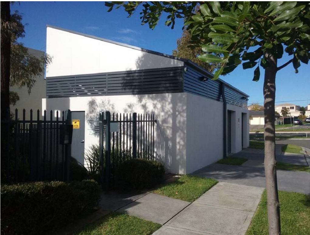
Photo of the same property as above after a screened bin and bulky waste storage area was built. (Photo: Blacktown City Council)
