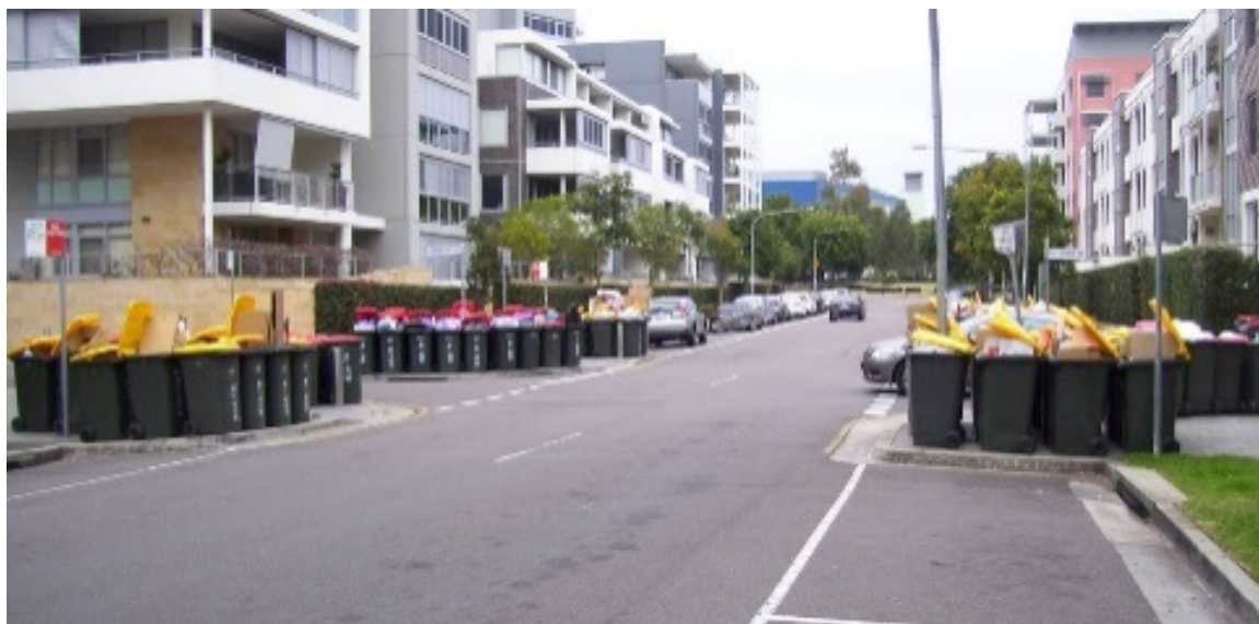
Bins serviced from the kerbside reducing public amenity and causing traffic hazards
