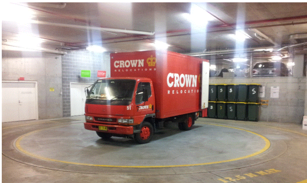
Example of vehicle turntable (Photo: Jacobs)
