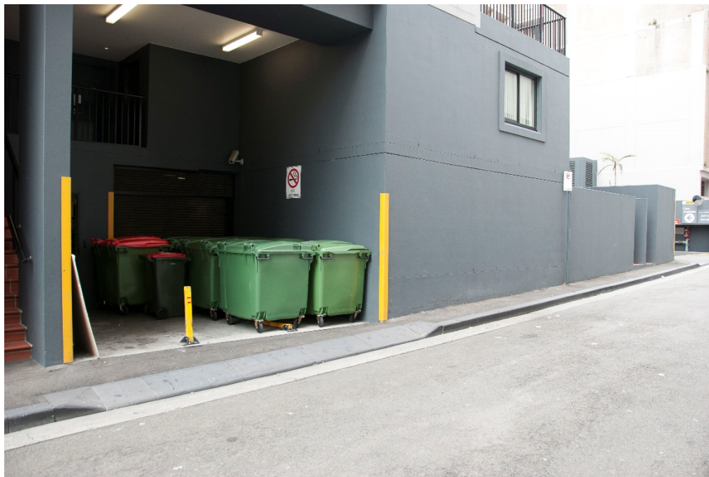
Collection point in the loading dock at rear of the mixed-use development Photo: Andrew Quinn
