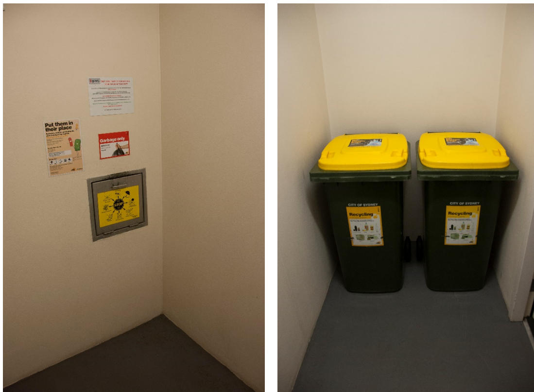
Bin storage and service rooms on each floor containing the chute hopper and two recycling bins in a mixed-use development. Photo: Andrew Quinn
