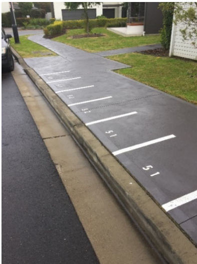
Good practice example of clearly defined waste service collection points for bin (Photo: Penrith City Council)
