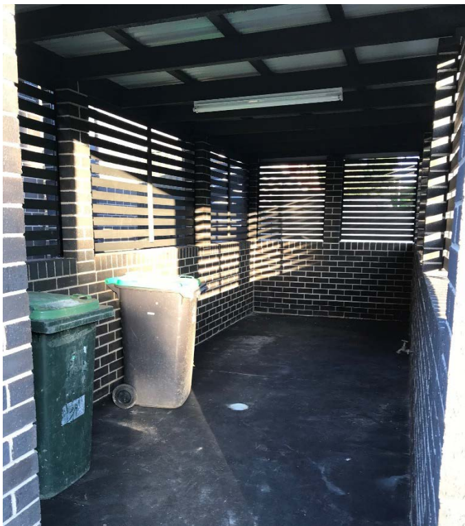
Bin storage with screening, robust construction and washing facilities (Photo: Penrith City Council)
