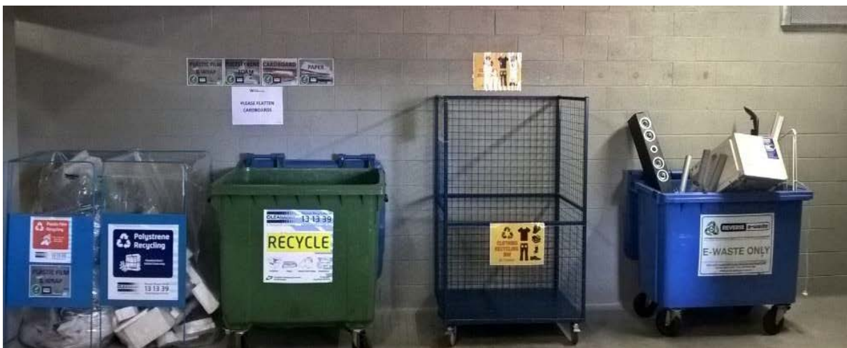
Problem waste storage area for e-waste, polystyrene, clothing and recyclables in the basement of a high-rise building – (Photo: City of Canterbury Bankstown)
