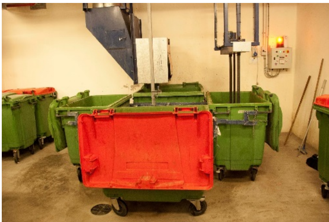
Four 660L bins underneath a waste chute with a ceiling-mounted compactor with bins rotated manually by the cleaner (Photo: Andrew Quinn)
