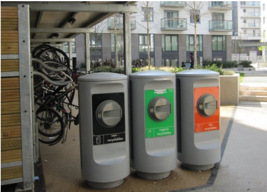
First AWCS installed in Australia (Photo: Sunshine Coast Council)
