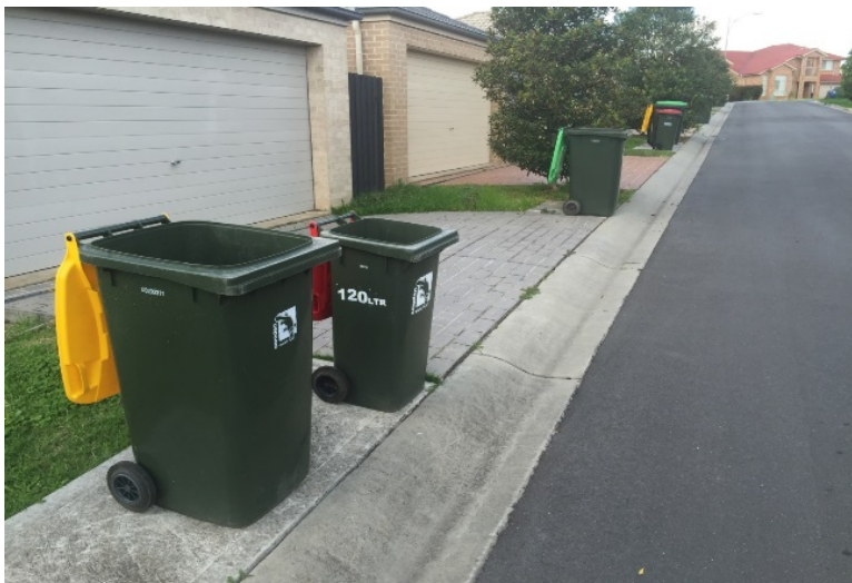
Bin pad made from concrete (Photo: Karina Maloney, Camden Council)
