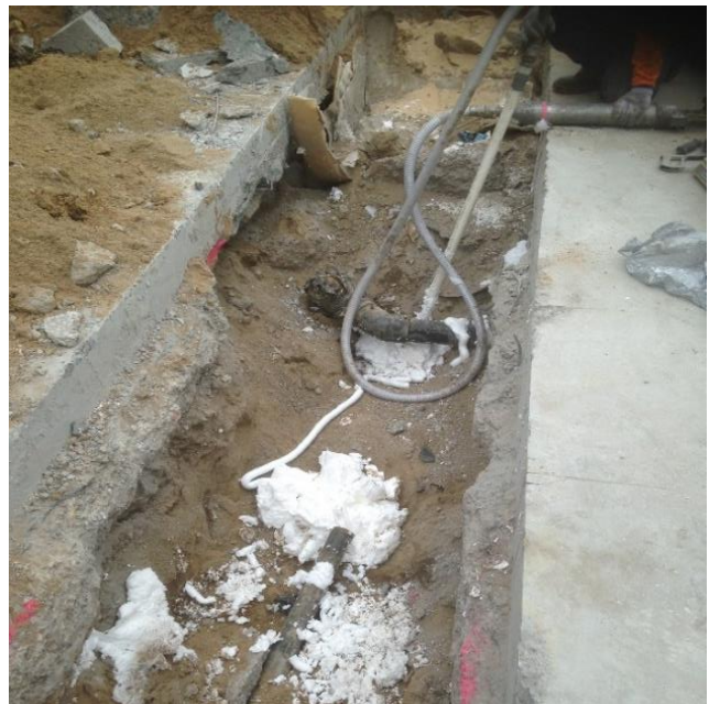
Decommissioning a storage tank in-situ by filling it with inert foam.
