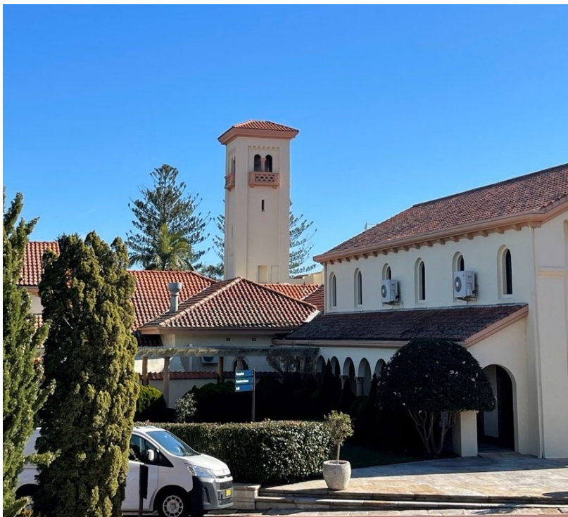
Figure 3 A well-designed stack with good height and conforming visually with the surrounding buildings
