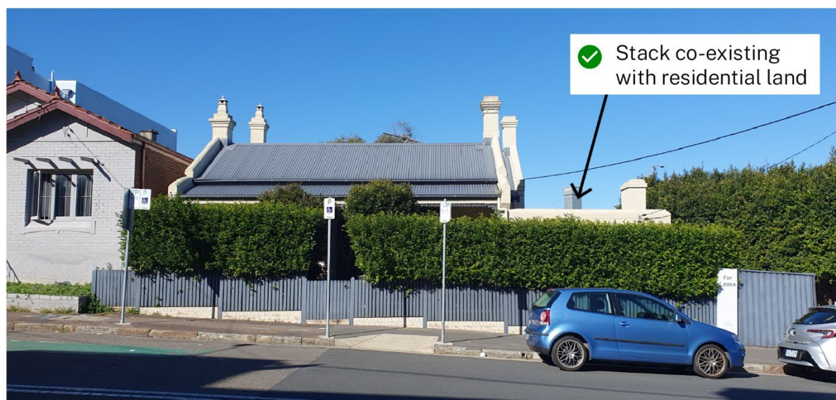
Figure 3 Stack visible above the roof line of nearby residential buildings
