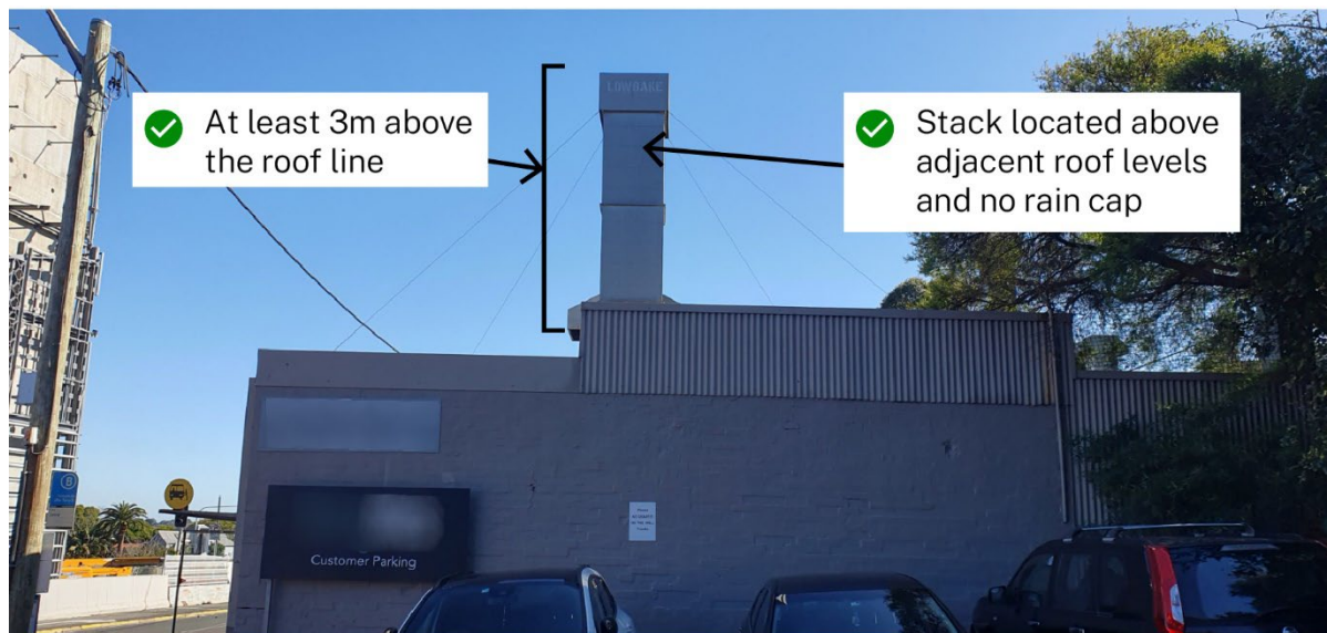
Figure 2 Well designed stack above the roof line of nearby buildings
