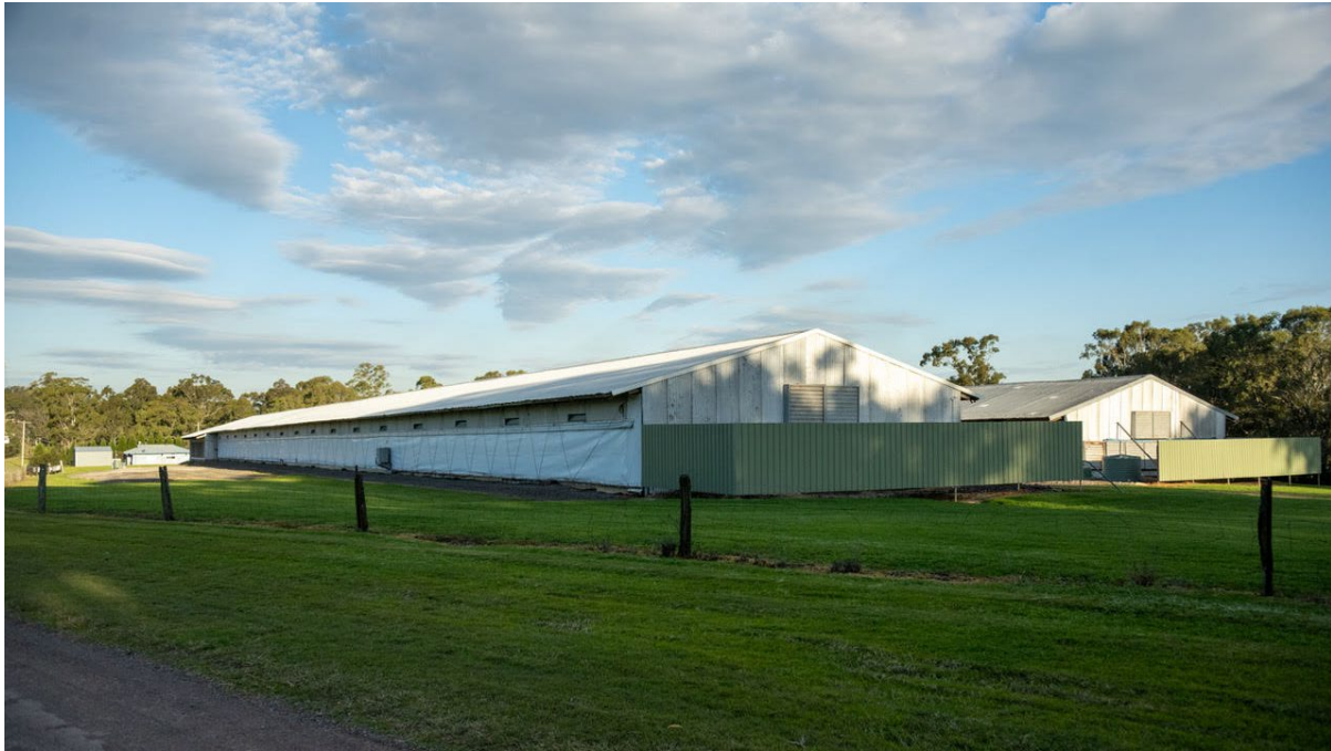
Figure 5 Example of a windbreak wall at the end of a chicken shed
