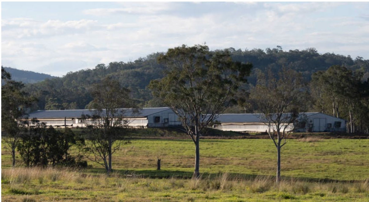
Figure 3 Example of ventilation outlets at the end of the chicken shed
