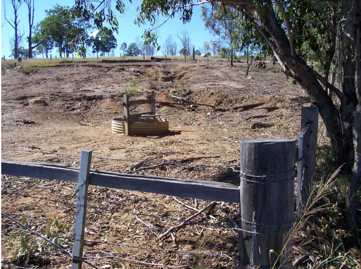
Photo 10 Severely eroded water point at base of Walloon Forest lands.
