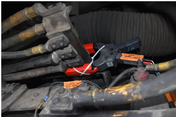
Current transducer on main AC alternator
