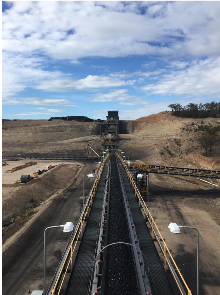
Figure 25 View along conveyor to ROM bin at MCCM
