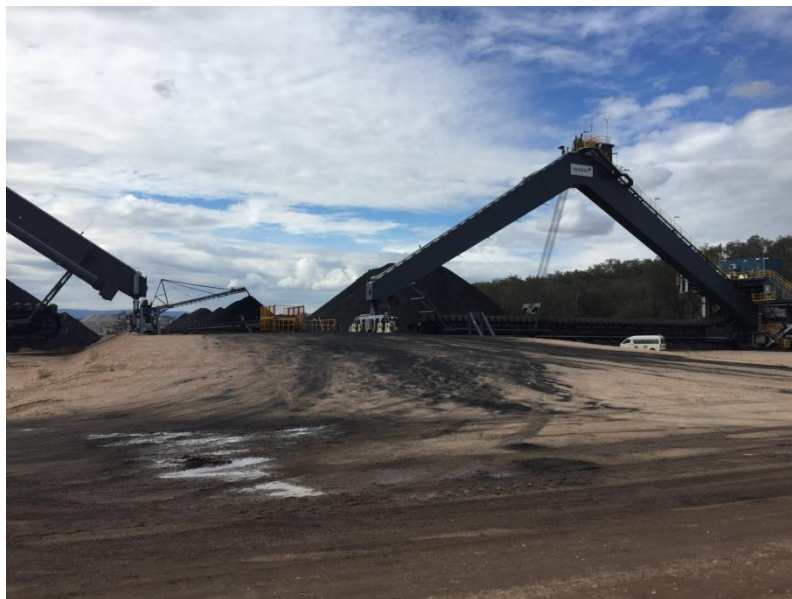
Figure 26 Portal reclaimer on product stockpile at MCCM
