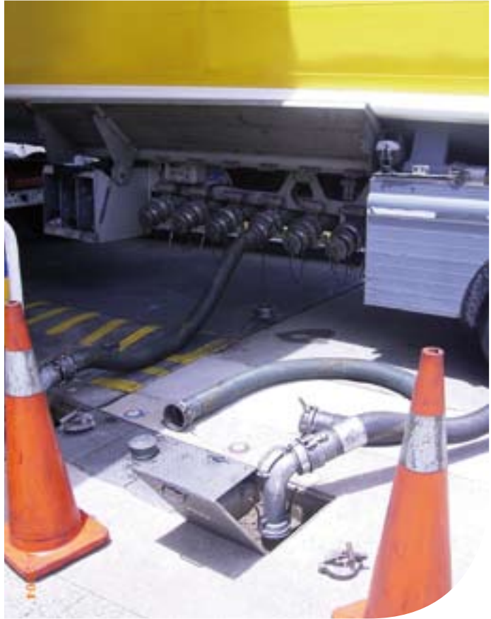
Road tanker connected to two hoses, one for pouring petrol into storage tank, the other for capturing vapours that are returned to the tanker.
