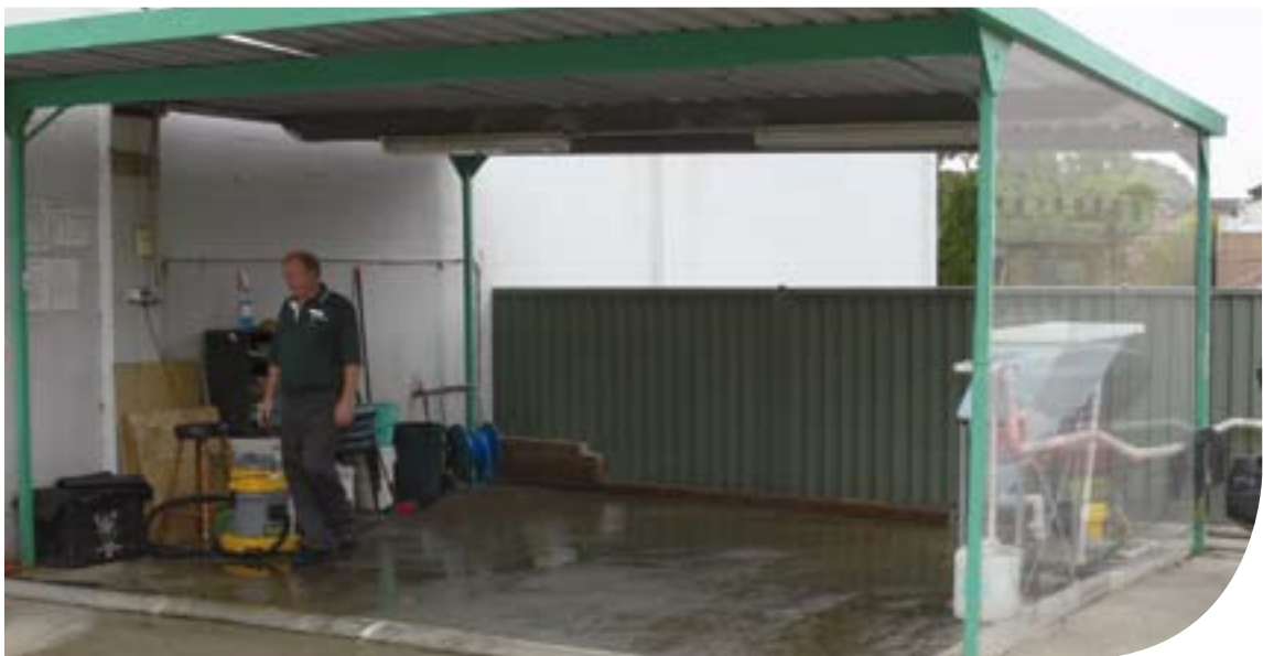
Wash area must be bunded and roofed.
