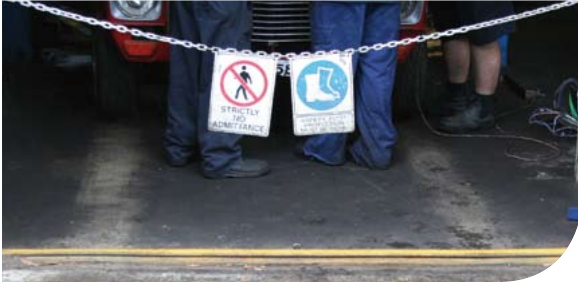
Workshop with drive-over bund.
