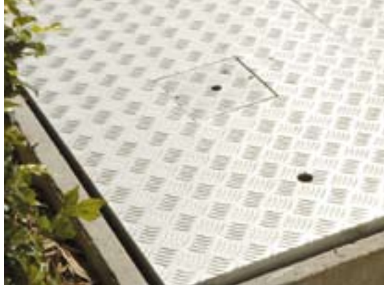
Ensure contaminated water from the forecourt is disposed of legally.
